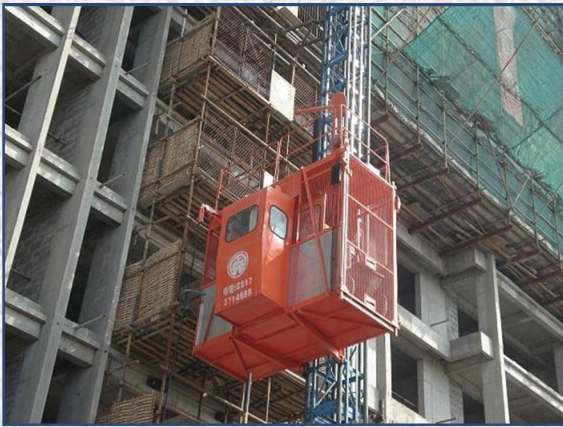
Construction elevator
