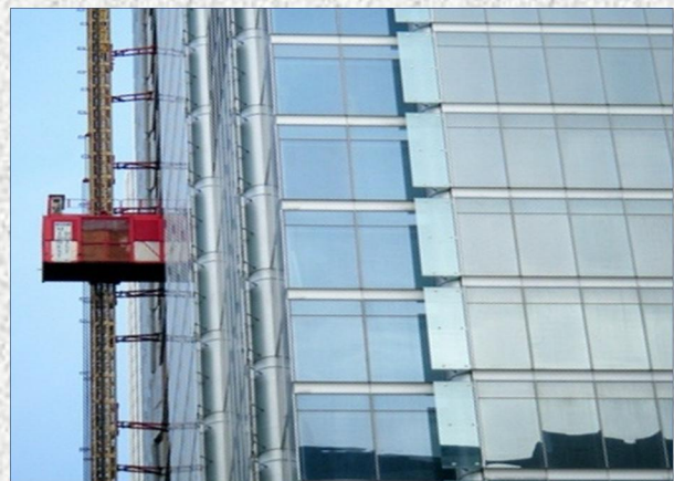
Temporary roof service hoist
