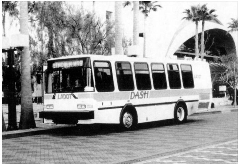
*Bus with microturbine hybrid-electric drive system*
