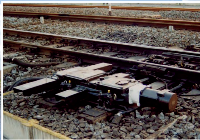
Railroad track switch with PHT 70
