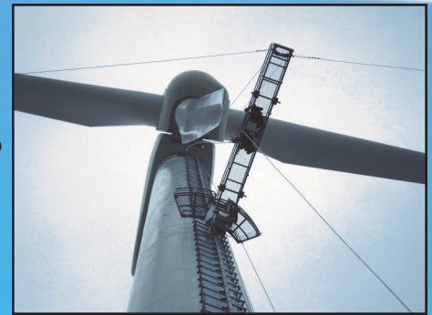
Bottom view of elevator with inspection basket lowered
